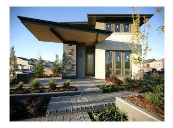
One of the most distinctive features that conveys the style is at the intersection of the roof and walls. The roofline can be flush, with a parapet, or dramatically overhang an entry or court. Broad overhangs provide shade, to help keep the home cool in summer months. These large overhangs are often cantilevered.
